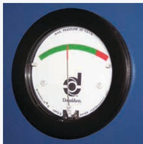
Differential pressure gauge(s) identifies filter maintenance.
