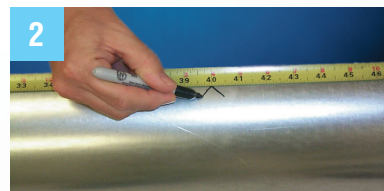
Mark distance to be spanned less 4".
