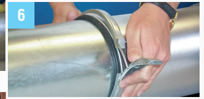
Snap clamp over O-ring and one end of nipple.
