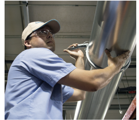
QF clamps together in seconds without welds, bolts, screws, flanges, special tools, precise measurements or specialized skills.
