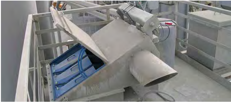
CPV - Pneumatically Filled Storage Bin 1,200 cfm (2,038 m³/h)
