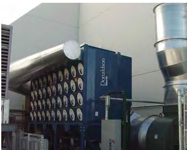
DWS on Custom Hand Grinding 38,500 cfm (65,398 m³/h)
