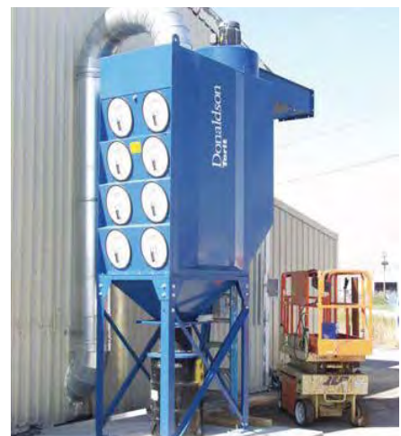
DFO on Plasma Cutting 5,000 cfm (8,493 m³/h)
