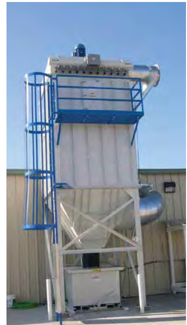
FS on Woodworking 20,000 cfm (33,973 m 3 /h)
