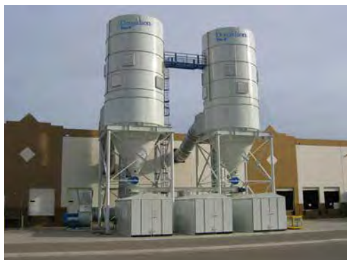
LP on Wood Dust 160,000 cfm (271,784 m 3 /h)
