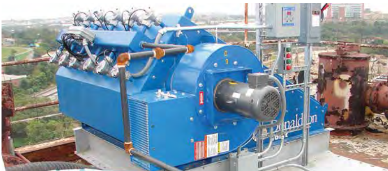
CPV - Multiple Cement Silos 4,800 cfm (8,154 m³/h)
