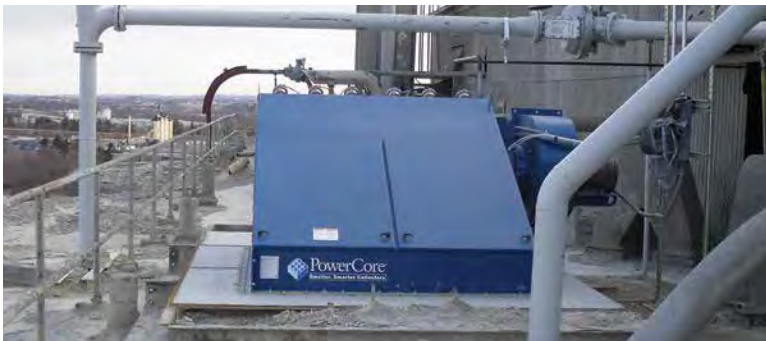
CPV - Multiple Cement Silos 4,800 cfm (8,154 m³/h)
