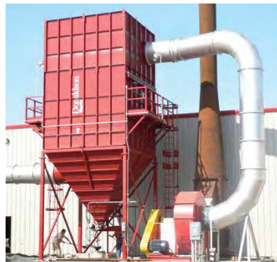
MB on Glass Processing 25,000 cfm (42,466 m 3 /h)
